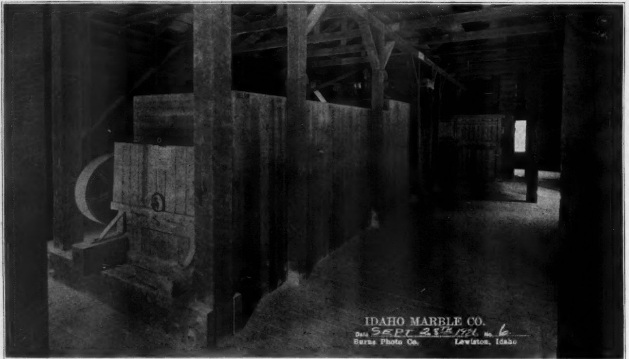
Interior Mill View. Note the Light and Clean Appearance
